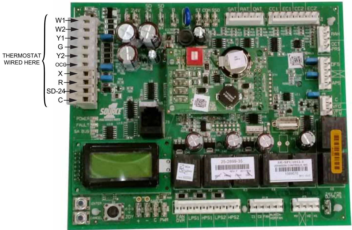
Figure 17: Unit Control Board
